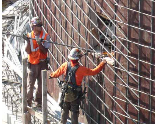
(IMAGE COURTESY OF KING COUNTY) DIGESTERS
