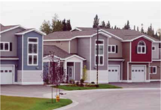
(IMAGE COURTESY OF NEESER CONSTRUCTION)
