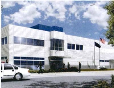
Photo: KPB ARCHITECTS/NEESER Goose Creek Correctional Center
