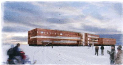
Photo: KUMIN ASSOCIATES/MAHLUM Norton Sound Regional Hospital
